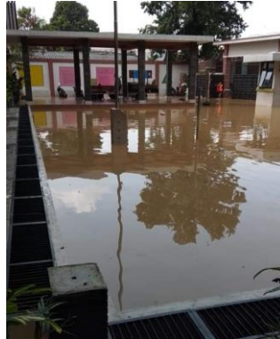
Figure 4. Floods at State Elementary school 05 Bidara Cina
