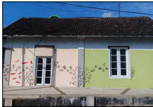
Figure 4. Building 2 (North) Side View (Personal Documentation, 2020)
