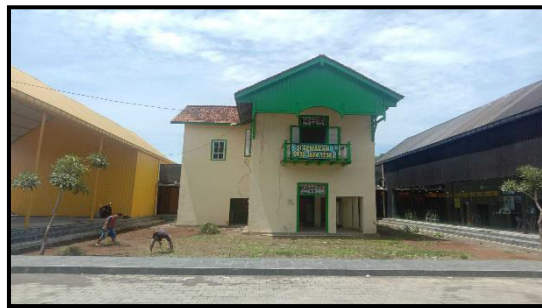
Figure 5. Differences Between Buildings On The North Side After Being Restored To The Ground. New Superstructure And Old Substructure (Personal Documentation, 2023)
