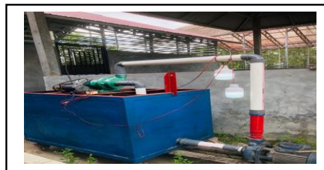
Figure 4. PAT Test with 30 Watt Load
