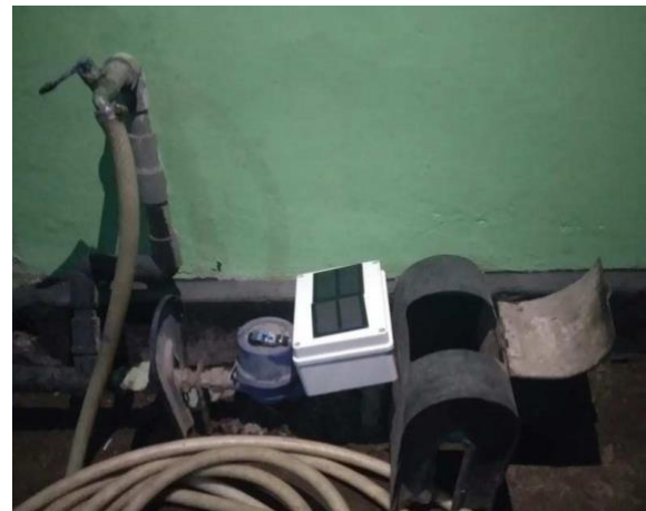
Figure 13. Implementation of a digital water meter reading system
